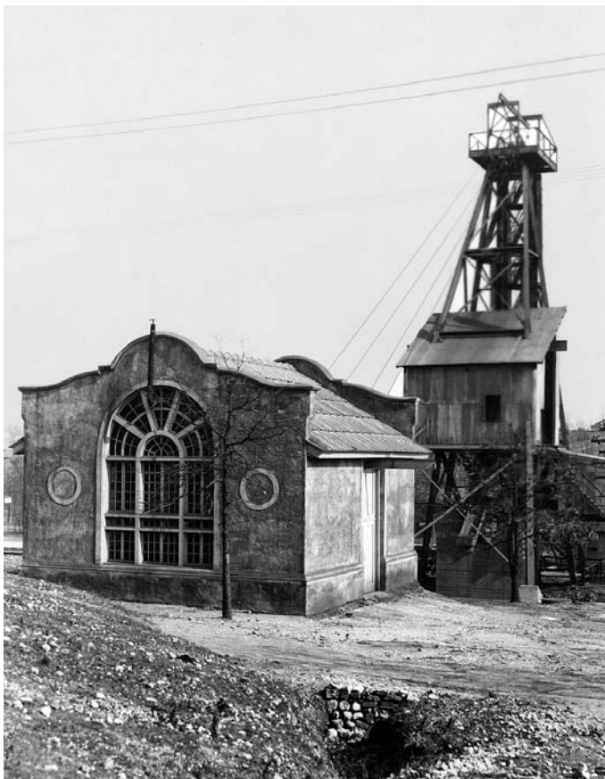
Woodward Iron Co., Redding Shaft Mine Hoist House, 1917-1927.
