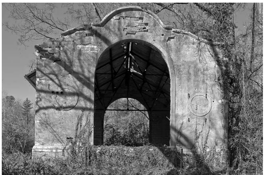
The Redding Shaft Mine Hoist House, 2009.
