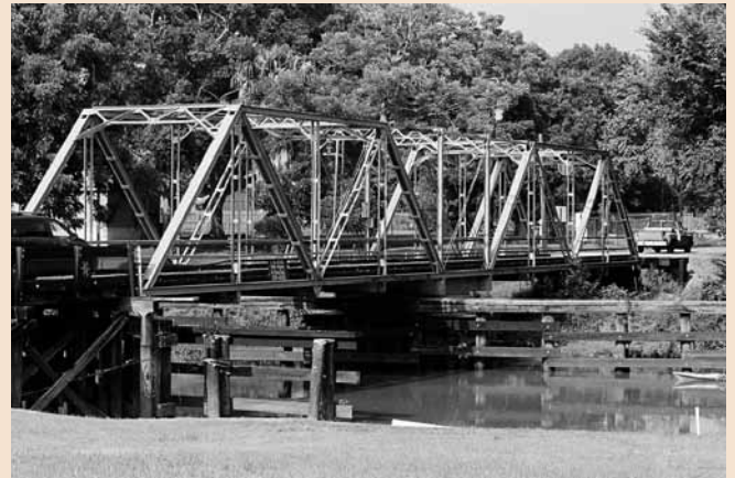
Swing-span bridge in Vida, La.
