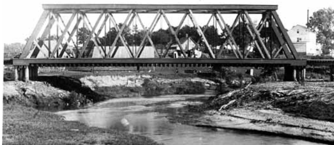
Railroad bridge, a Howe with sloped end posts. Danbury, Iowa.
