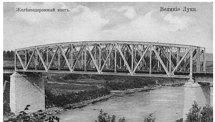
Warren truss with vertical ends. Examples in the U.S. are very rare; this example is located in Russia.
