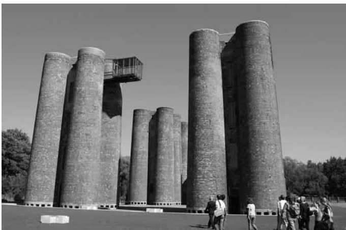
Biotowers in Lauchhammer.
