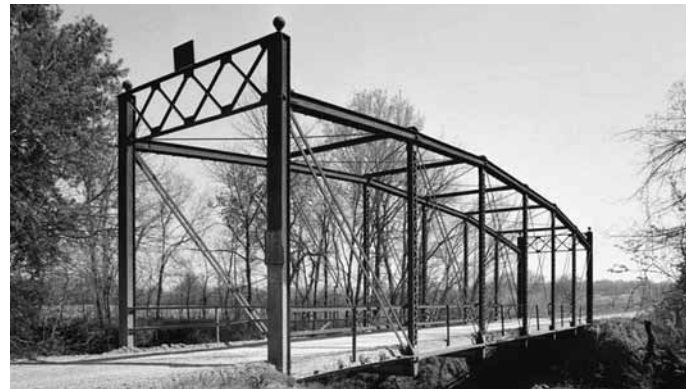
Onion Creek Bridge, Coffeyville, Kan., a Pratt with vertical end.
