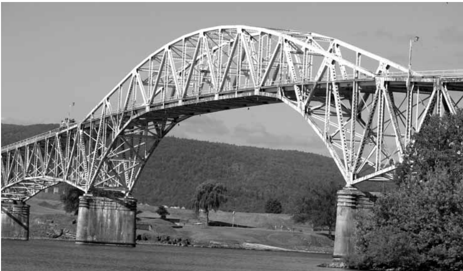
The Lake Champlain Bridge, a nationally significant example of continuous-cantilever truss design, was demolished in December 2009.
