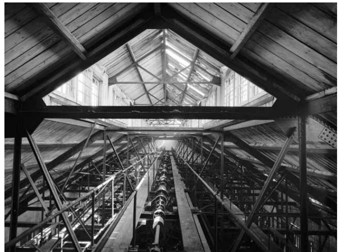
Jet Lowe, Photographer, July 1978. Central line shaft and roof trussing in 1900 Machine Shop.
