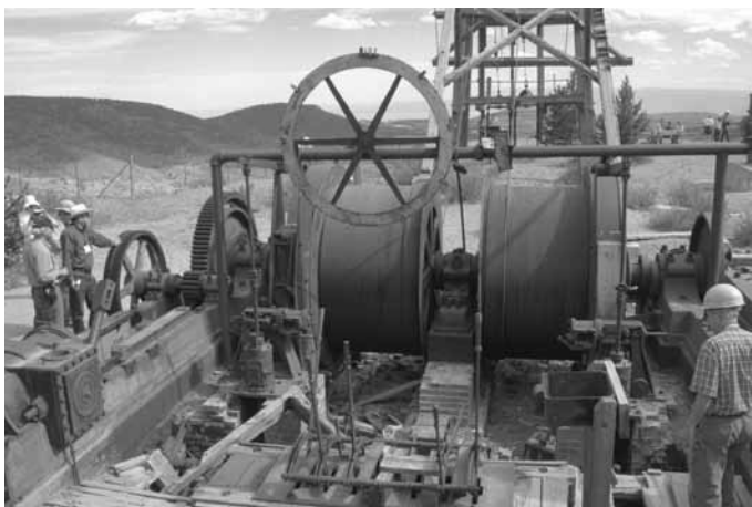
The hoisting engine at the American Eagle Mine.
