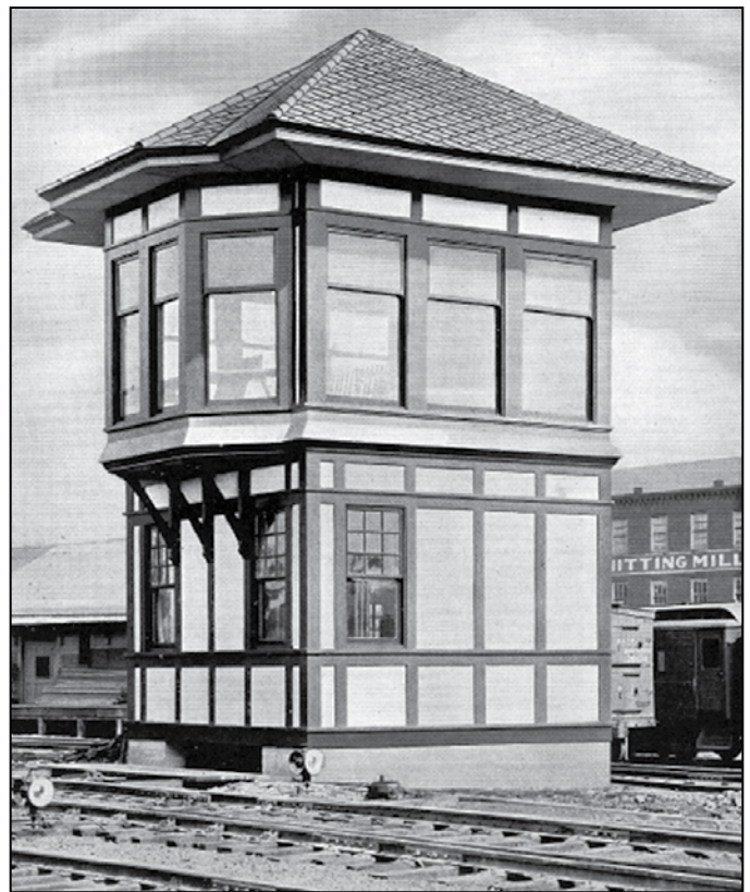
Railroad structure roofed with ASS&S shingles (ASS&S 1922).
