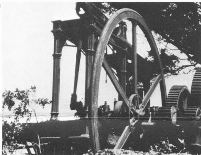
(l) The West Point beam engine & drive gearing to mill. (r) Side view of the three-roll cane crushing mill.
