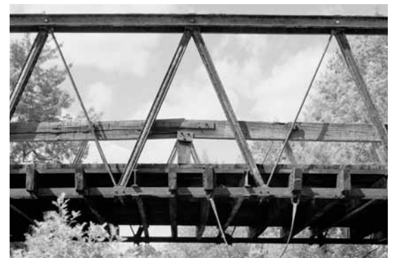
Phoenix columns enclose tension rods at mid-span of the Atherton Bridge.
