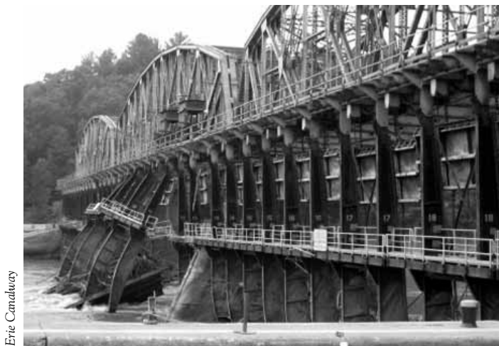
Steel uprights at Lock 11 on the N.Y. State Barge Canal were forced out of position by rushing water and debris.
