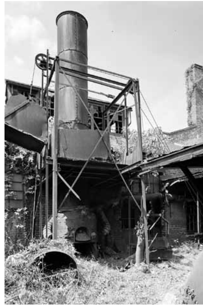
The cupola furnace at the Appomattox Iron Works, Petersburg, Va.
