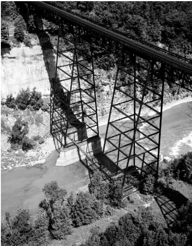
Portage Viaduct, HAER NY-54 (1971).
