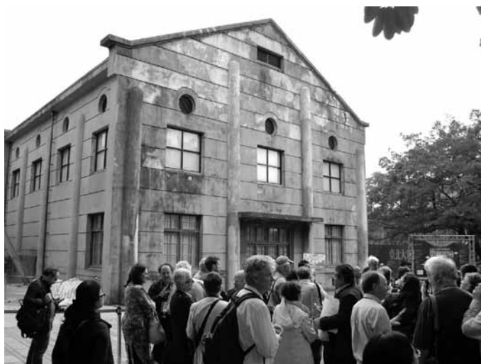
Songshan Tobacco Factory powerhouse.
