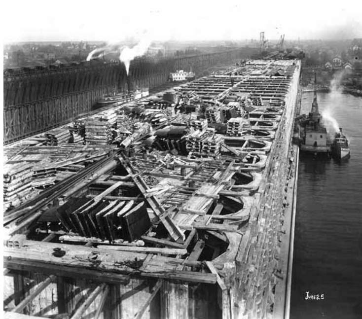
Construction of the Ashland Ore Dock, June 25, 1917.
