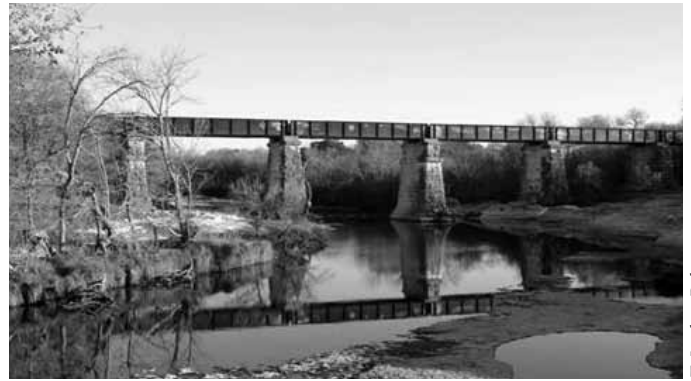
Nolan River Bridge. T. Lindsay Baker
