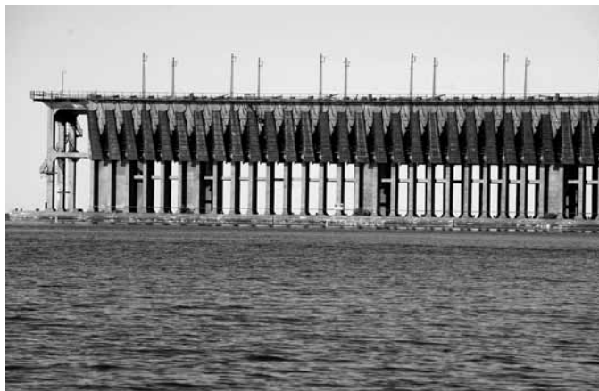
Ashland Ore Dock in 2012.
