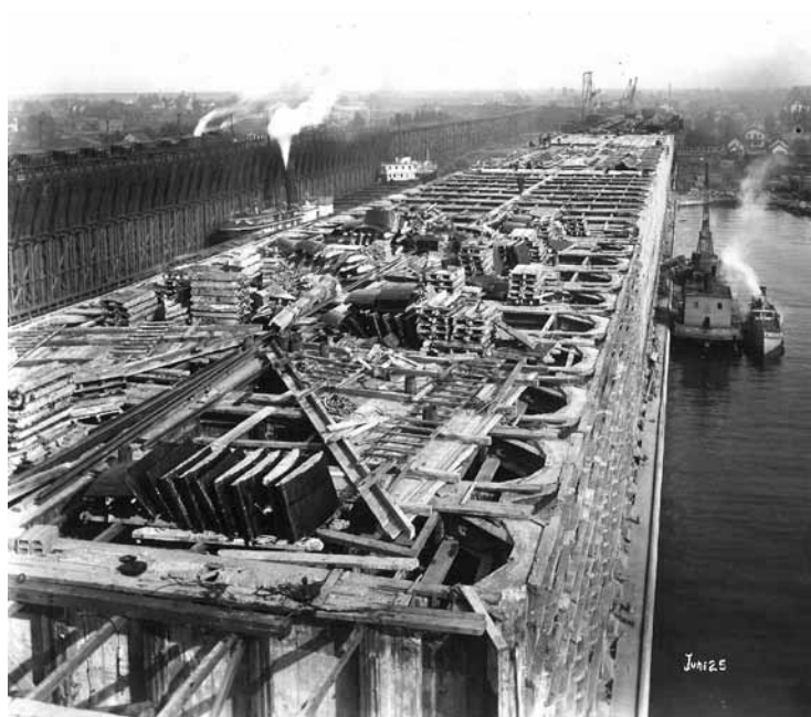
Construction of the Ashland Ore Dock, June 25, 1917.
