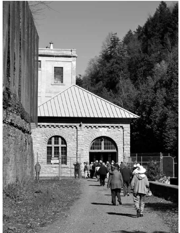
Trenton Falls hydroelectric plant.
