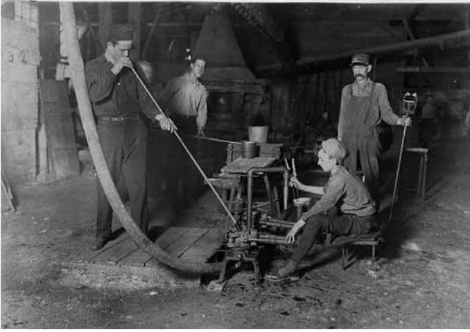
Blowing hollowware at a glassworks in Grafton, W.Va., 1908. The tongs in the mold boy's right hand appear identical to those recovered at Glassboro. Note the shim beneath the mold's left leg, likely inserted to steady the mold on an uneven floor; the iron wedge recovered at Glassboro may have served the same purpose. This scene likely compares well with operations at the Whitney Glass Works, circa 1900.
