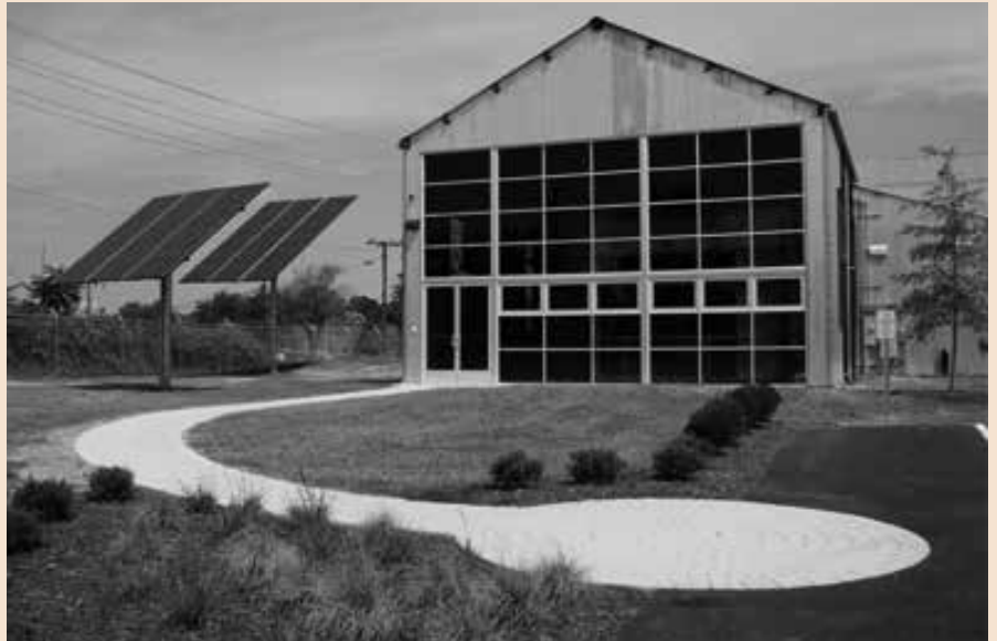
The renovated car barn of the R&CB in Richmond, Va.
