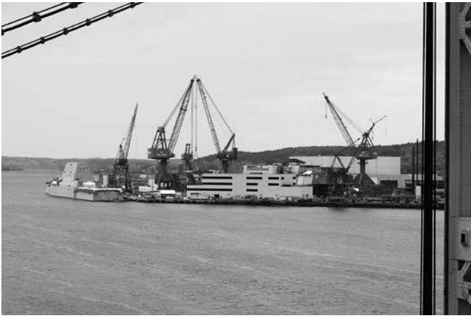
Bath Iron Works from the Carlton Bridge.
