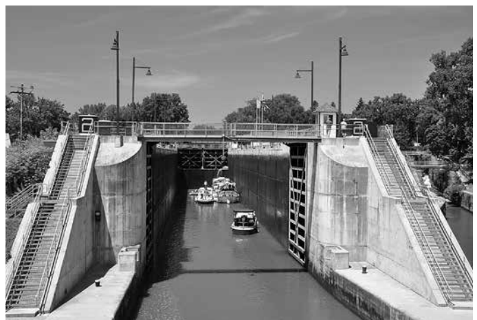
New York Barge Canal, Lock E2, Waterford, N.Y.
