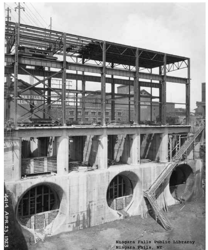
The Niagara Falls (N.Y.) Public Library is seeking assistance dating and identifying the technological features and perhaps some of the individuals depicted by this set of four photos, part of a much larger collection held by the library. The massive riveted control valve (disc) is thought to be a headgate for the penstock on the Upper Niagara River above the Schoellkopf Generating Station. Info: William H. Seiner, whseiner@gmail.com , (716) 876-7340.
