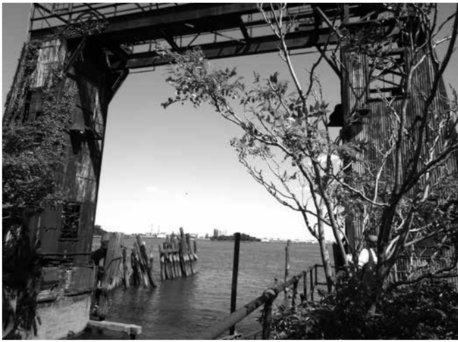
134th St. Ferry Bridge, view looking east into the East River.
