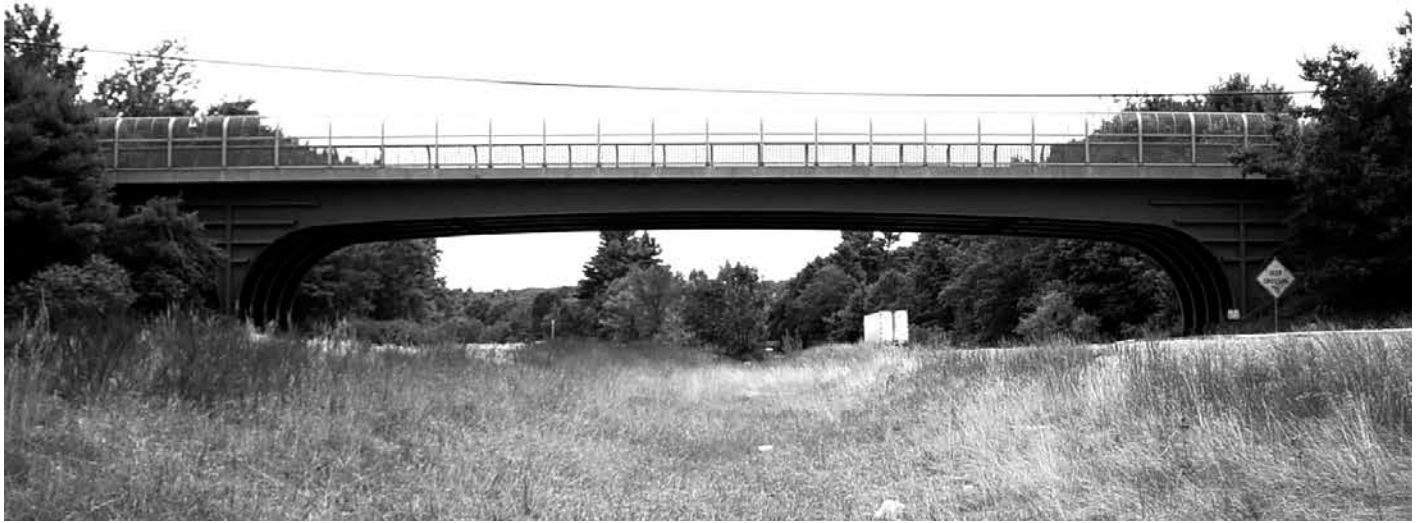
Robert J. Prowse Memorial Bridge (Ash St. over I-93).
