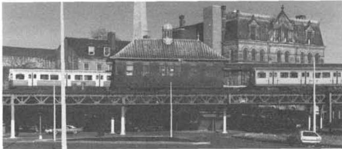
Thompson Square Station, 1901, before removal from the Elevated structure. Richard J. Brillante photograph.
