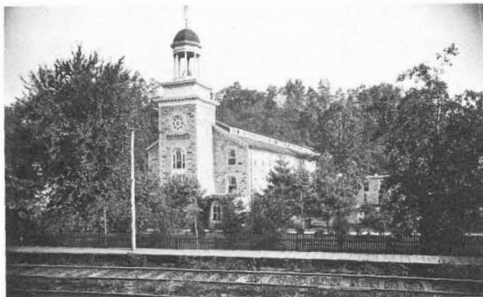
Alberton Mill, c1870, and as the Daniels Mill, 1968, the housing partially demolished (lower left).
