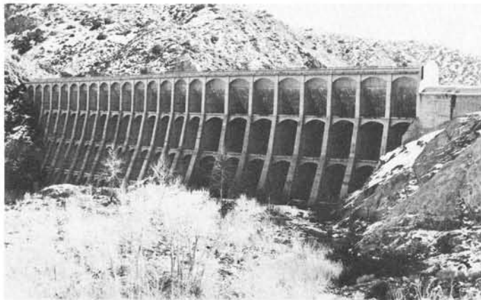
LITTLEROCK DAM, 1924. (L) Buttresses on the downstream side, 24 feet on center, create a "hollow dam." Spillway is at far right. (R) The upstream face consists of 29 arches angled at 45°, supported by the buttresses. Spillway is in the foreground. Donald C. Jackson photographs for HAER.
