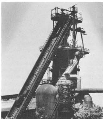
SLOSS FURNACE, skip hoists for charging in foreground. Historic American Engineering Record photograph.
