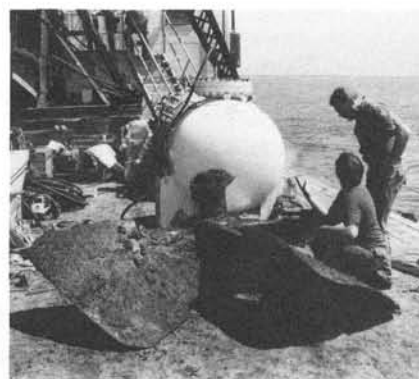
Indiana's engine and boiler greeting the light of day for the first time in 121 years. At right is the vessel's Ericsson-type composite propeller, with cast-iron hub and wrought-iron-plate blades, one of them stamped with the name of Spang & Co., Pittsburgh, rollers of the iron. This was the only marking found on the elements raised. National Museum of History & Technology photographs.
