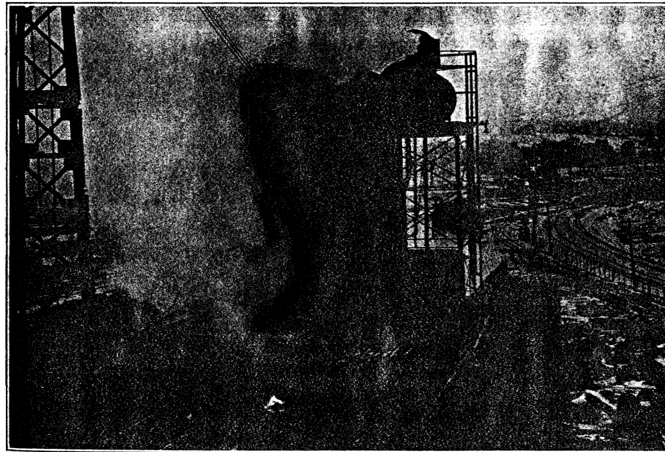
Figure 4.—One of the quenching stations in operation. The side walls serve as a stack, and carry most of the steam up and away from the quenching-car operator.
